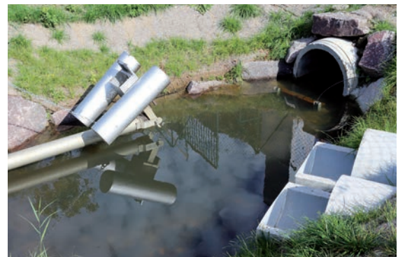
Rain water treatment unit in Ostwald
