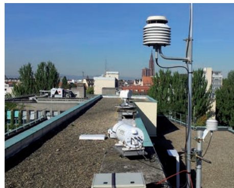
Climate monitoring unit
